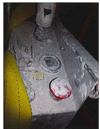
Equipment is inspected
