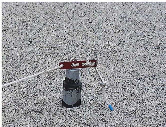
Only one item tied back to roof anchors
