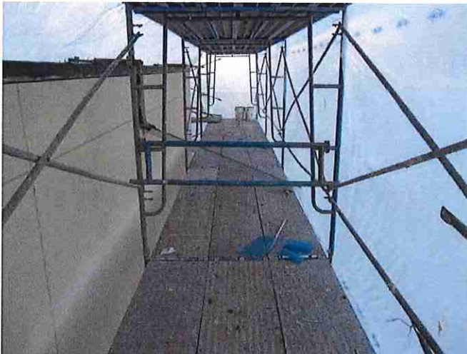
Block off areas that are not complete
