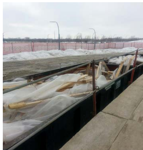
Place wet material in container to later dispose of into jobsite dumpster.
