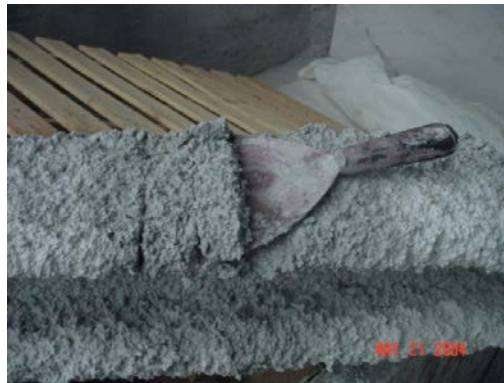
Scrape off wet material with tapping knife
