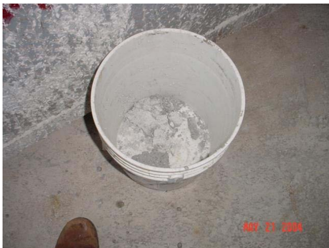
Place wet material in container to later dispose of into jobsite dumpster.
