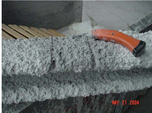
Score wet material with a utility knife
