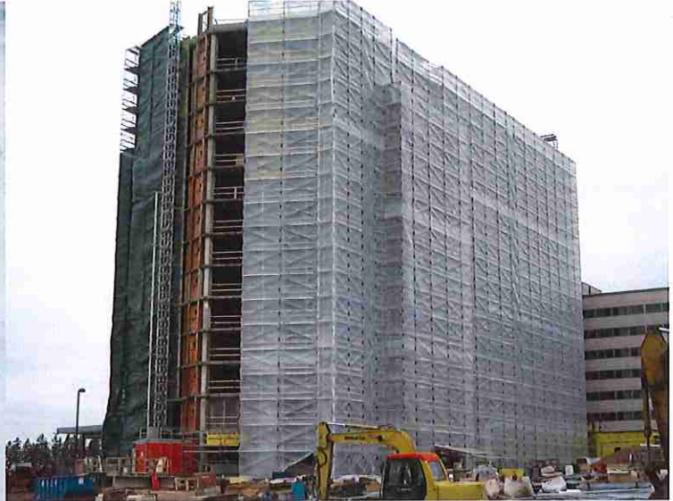
Temp heat & additional scaffold tie ins.
