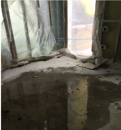
Cause of Mold: (warm/wet conditions inside the building)
