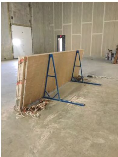
PREVENTION: (keep material off the floor, GC to dry out areas before stocking material)
