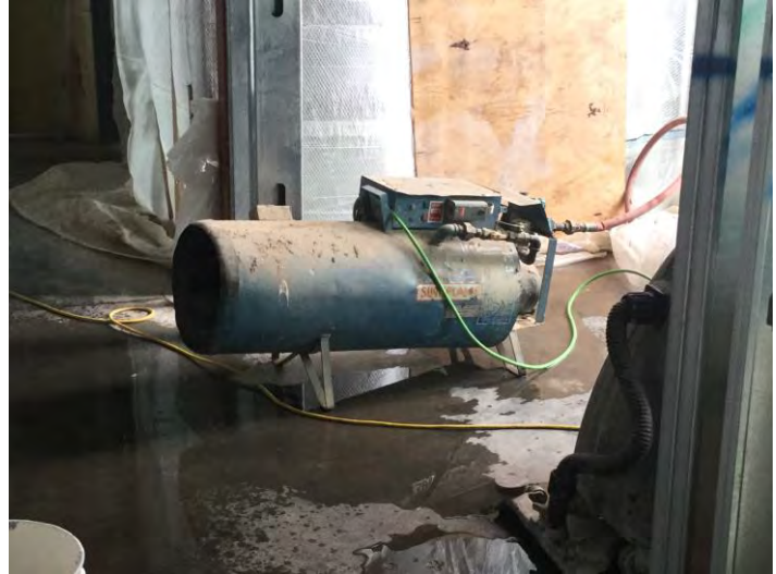
Cause of Mold: (warm/wet conditions inside the building)
